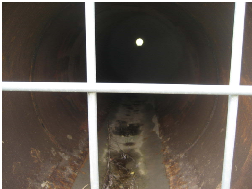
Figure 7.3 – Mammal tunnel under the A64 carriageway
