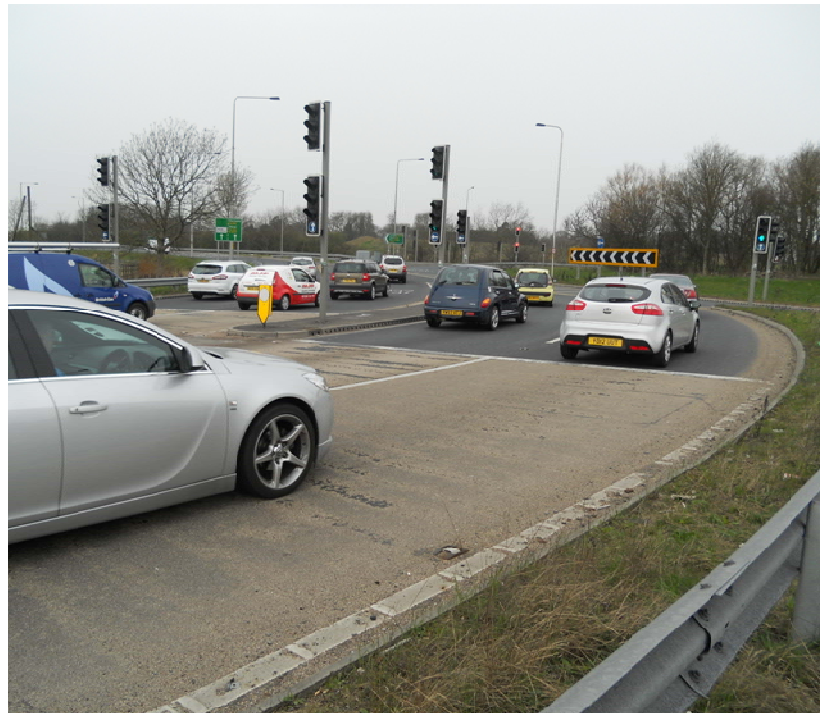
Figure 2.3 – A64 South approach showing widened carriageway and traffic signals
